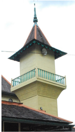
Gambar 7: Menara Masjid Kraton Sambas
